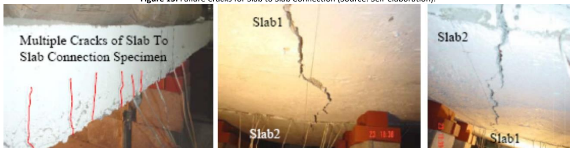
Figure 15. Failure Cracks for Slab to Slab Connection (Source: Self-elaboration).
