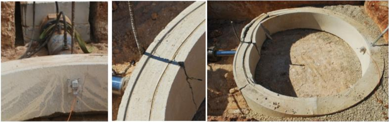
Figure 5. Pipe In situ tests. Source: Own elaboration (2018).
